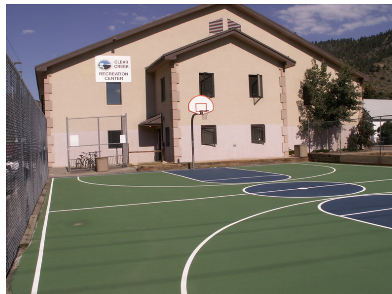
Figure 1: The Clear Creek Recreation Center in Idaho Springs is the flagship facility for the District.
