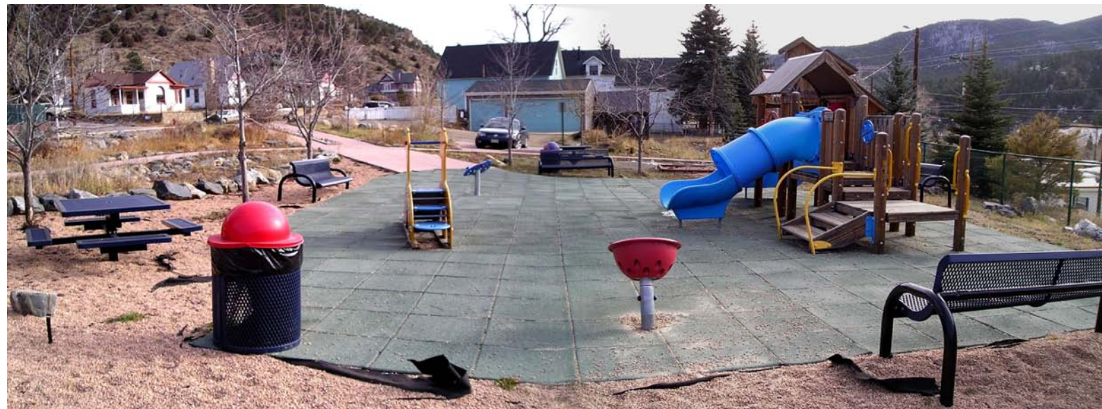
Figure 46: Safety surfacing at Macy/Ruth Mill Park needs to be refurbished.
