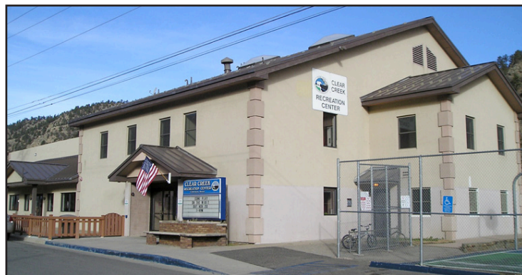
Figure 17: The Clear Creek Recreation Center is the central facility for the District.
